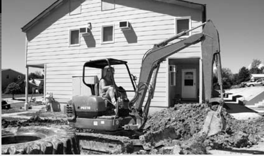
A Lind-Exco operator uses a Komatsu PC27R to dig a trench at a housing project in Rapid City. The company uses the PC27R on smaller projects where its larger excavators can't go.
