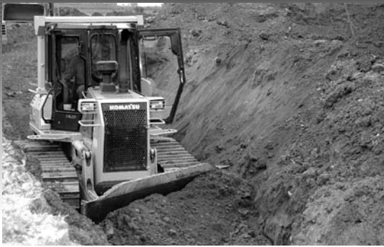
Grizzly Excavation often rents equipment from DMI, such as this D41 dozer used for backfilling a trench at a utility project in Box Elder.
