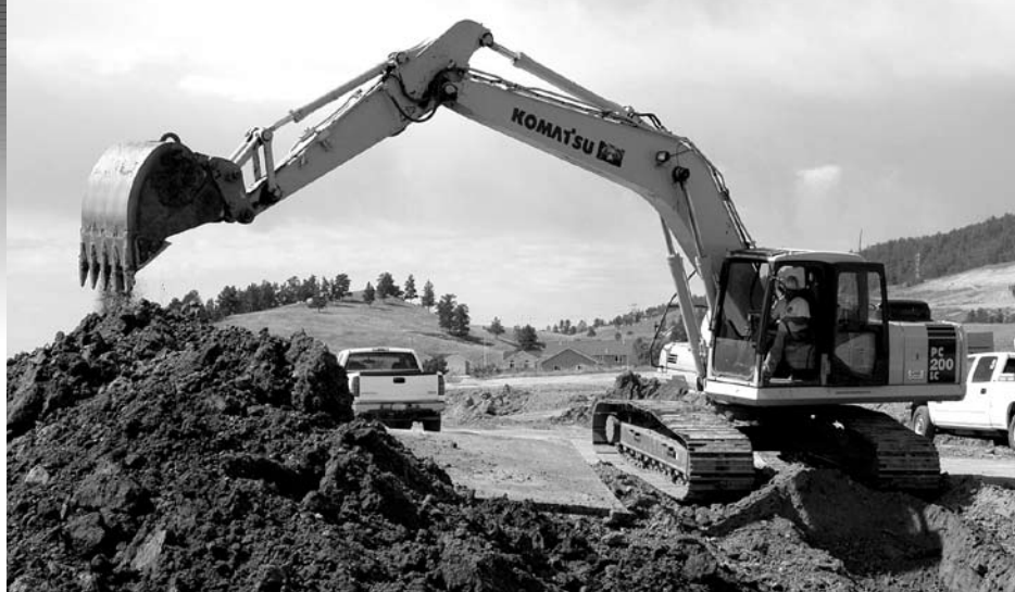
A Grizzly Excavation operator uses a Komatsu PC200LC-7 excavator to pile dirt from a trench at a utility project near Box Elder.
