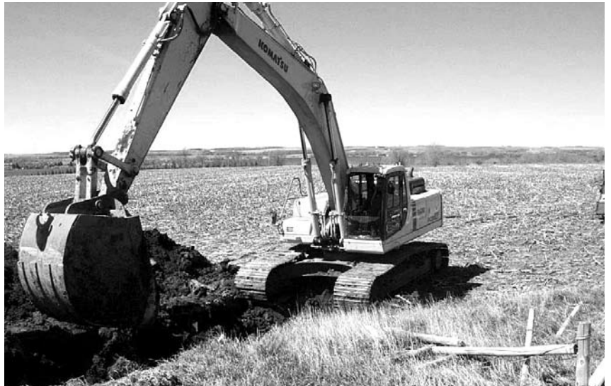
For deeper digs and larger pipe, Mark Mathieu Construction turns to its PC300LC-6 excavator, shown here digging a trench for a rural water line.
