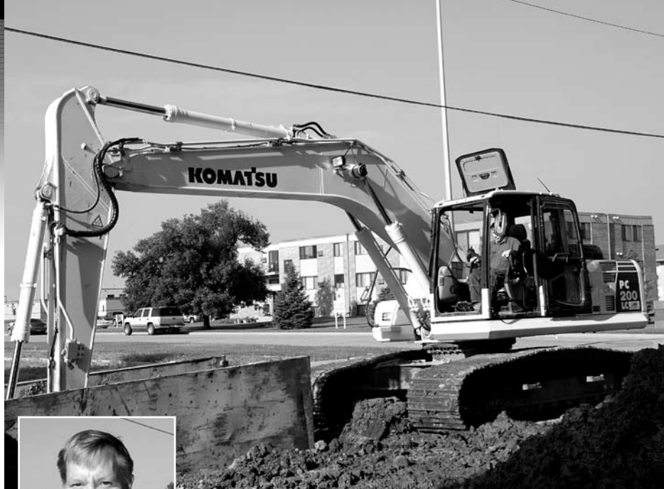
Using a Komatsu PC200LC-8, Supervisor Daryl Bellikka digs a trench for new water lines in Huron. The PC200LC-8 features a Tier 3 engine that offers less fuel consumption with more productivity. "There's a noticeable difference in the amount of fuel used," said Bellikka.
