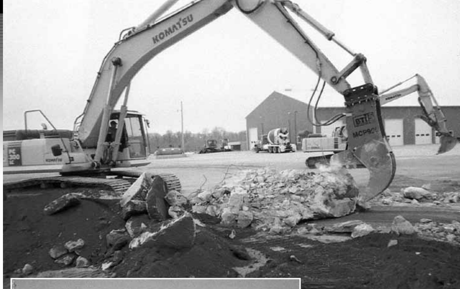
Valley Sand & Gravel, a sister company to Tri-State Ready Mix, used Komatsu excavators to break up old concrete in preparation for recycling it using a rented Komatsu BR380JG crusher.
