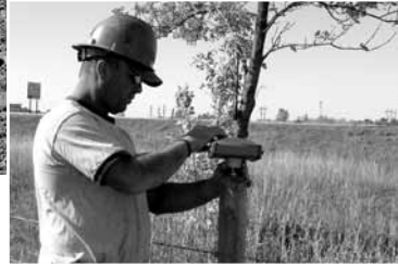
Brad Schoenfelder sets up a Topcon 3D-MC 2 base unit used to set grade via GPS with a Komatsu D51 dozer on a jobsite in Mitchell.
