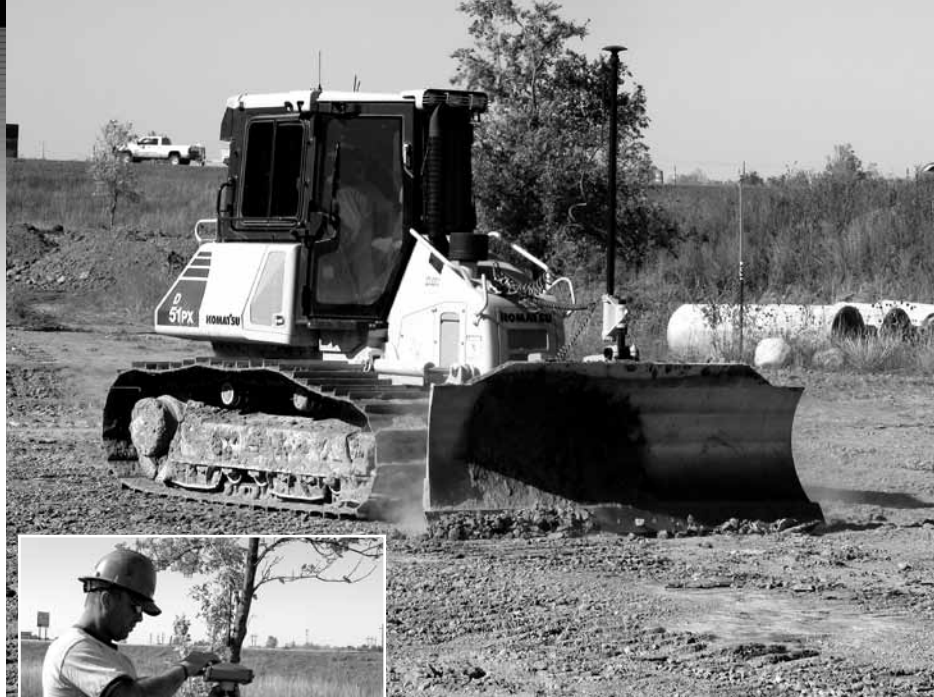
Brad Schoenfelder sets up a Topcon 3D-MC 2 base unit used to set grade via GPS with a Komatsu D51 dozer on a jobsite in Mitchell.
