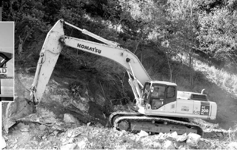
This Loiseau Construction operator uses a Komatsu PC300LC-7 excavator to remove rock in preparation for road widening on Highway 52 near Yankton, S.D.
