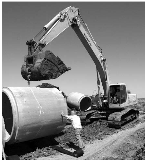
A Loiseau Construction operator uses a PC400LC-6 to excavate trenches and set pipe on the reconstruction of Highway 11 from Canton to Beresford.
