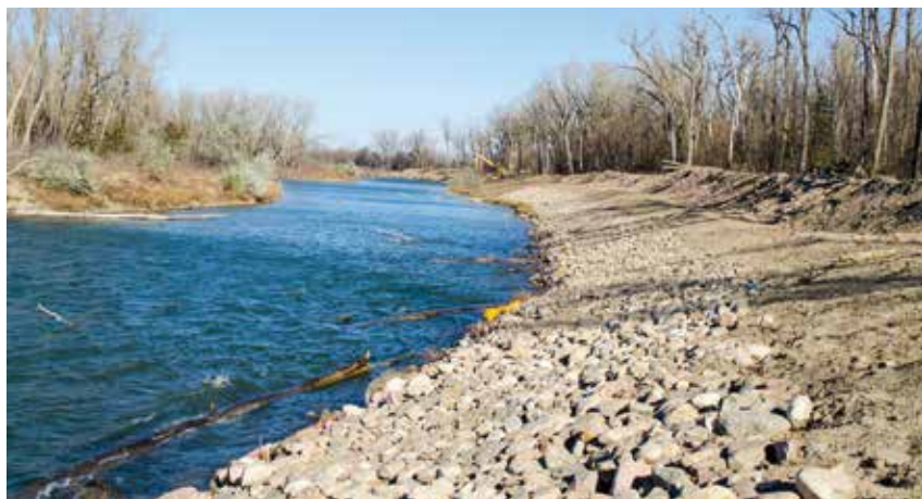
Quinn Construction completed a shoreline-protection project for the U.S. Army Corps of Engineers and the South Dakota Game, Fish and Parks Department in December. The company created and reinforced a slope that started four feet below the Missouri River and extended as high as 40 feet in some areas to protect the Lewis and Clark Water District's wells.
