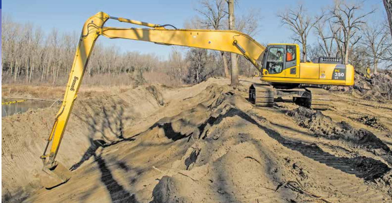
Field Superintendent Eddie Seieroe uses Quinn Construction's Komatsu PC350LC with a long stick to create an 80-foot, two-to-one slope along the Missouri River. "We needed the reach of the PC350LC to complete this job," said Seieroe. "At full extension, I still have excellent power and control. There is no jerking from the controls. It's a smooth machine."
